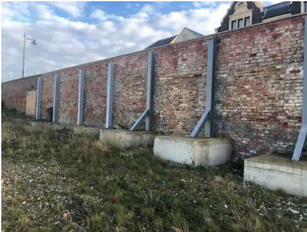
Plate 4: Supports for the facade of the former Staiths House
