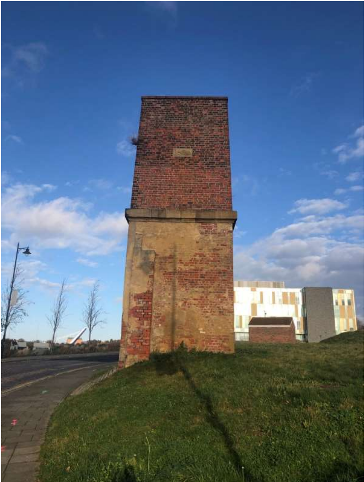
Plate 6: 1865 chimney from the south. The date stone can be seen mid-way up the unrendered top section
